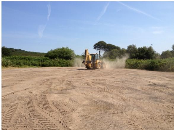
Work was also undertaken through scraping, the additional use of on-site material and rolling to improve existing car parking facilities at Four Firs, Estuary and Joney's Cross car parks, with maintenance of all barriers across the SSSI on-going. Works to improve track drainage was also undertaken on Dalditch plantation.
